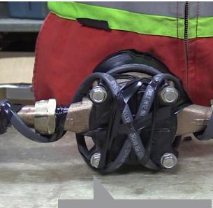
**PRO TIP! Apply the heat** trace in a cross-cross pattern under the water meter
