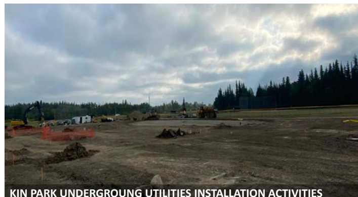
KIN PARK UNDERGROUND UTILITIES INSTALLATION ACTIVITIES
