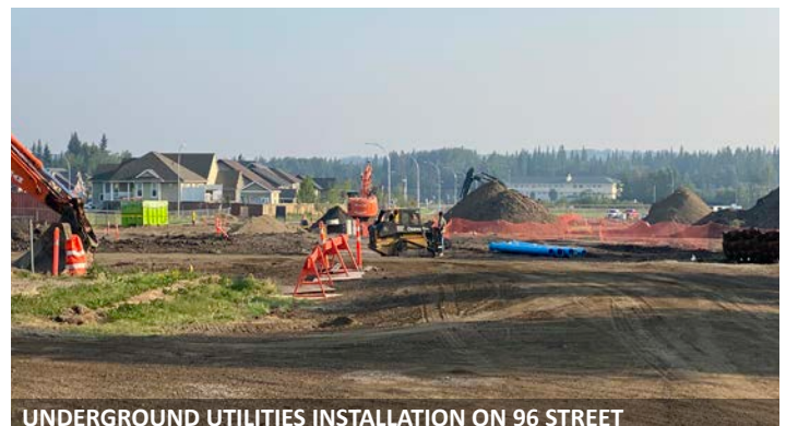
UNDERGROUND UTILITIES INSTALLATION ON 96 STREET
