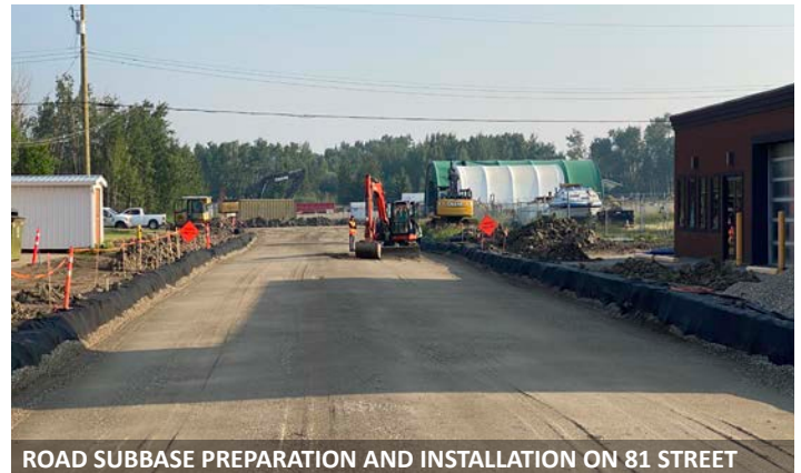
ROAD SUBBASE PREPARATION AND INSTALLATION ON 81 STREET
