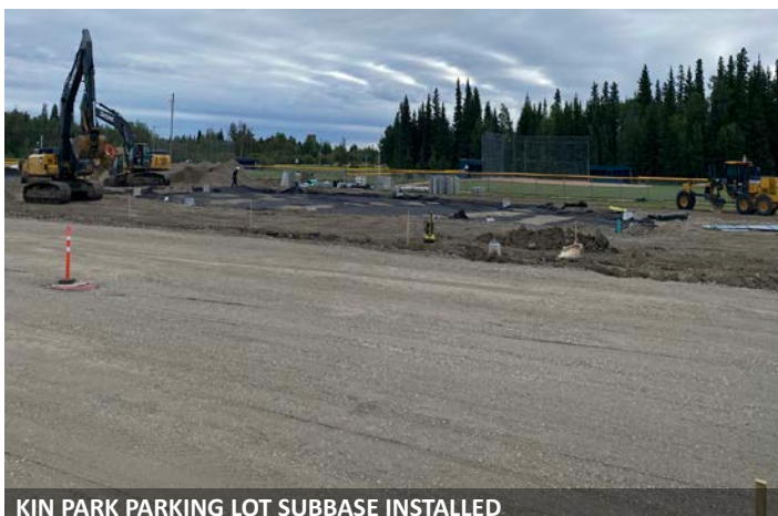
KIN PARK PARKING LOT SUBBASE INSTALLED
