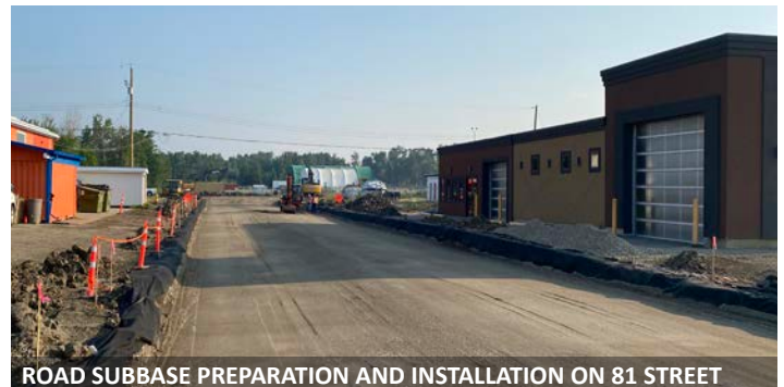
ROAD SUBBASE PREPARATION AND INSTALLATION ON 81 STREET
