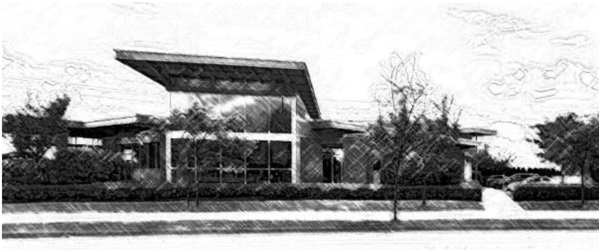
Figure 25: Building showing architectural detail
